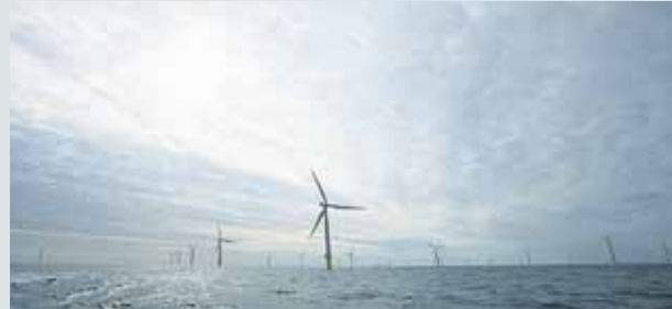
With 48 wind turbines and a transformer station out at sea, the Lillgrund offshore wind farm is one of the largest of its kind anywhere in the world.
